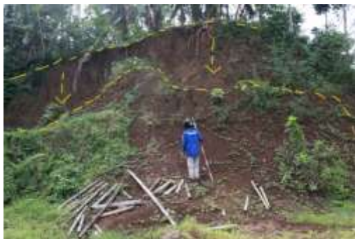
b. Landslide Type Topple at Plantation Area (UTM 49M X: 357406 Y: 9193567)
